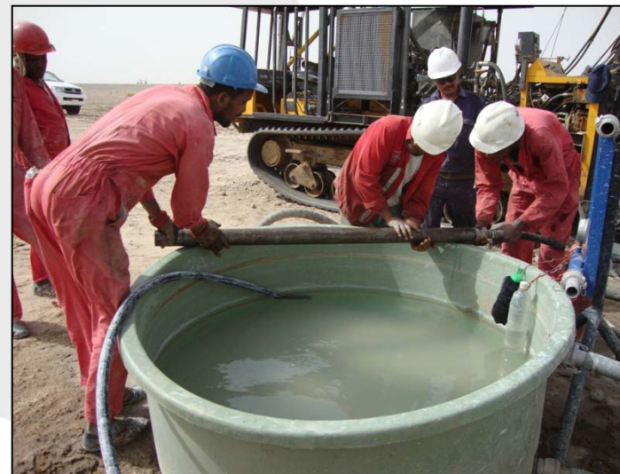
Diamond drilling at the Colluli Potash Project, Eritrea.
